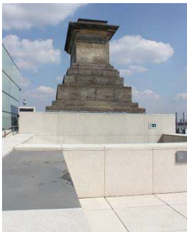
Fig. 4 Placement of new and historic elements next to each other
