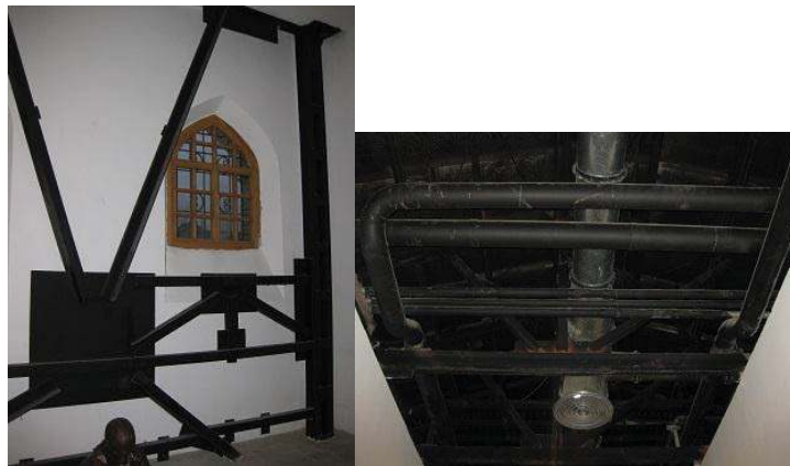
Figs. 48 and 49 Visible attached structure and installations
