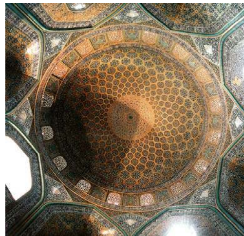
Fig. 3: Interior view of Sheikh Lotf-Allah Mosque dome (Noor Bakhtiar, 2001: 13)
