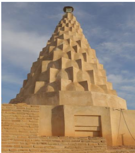
Fig.10. The chipped dome of the building
