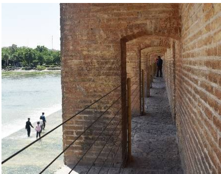
Fig. 1 Allahverdi Khan Bridge, a covered corridor on both sides of the bridge overlooking the river
