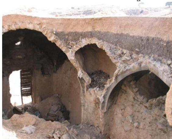
Fig.22. Layers of covering between the arch and the roof in one of the villages of Shushtar city (Chaharmahali, 2016)
