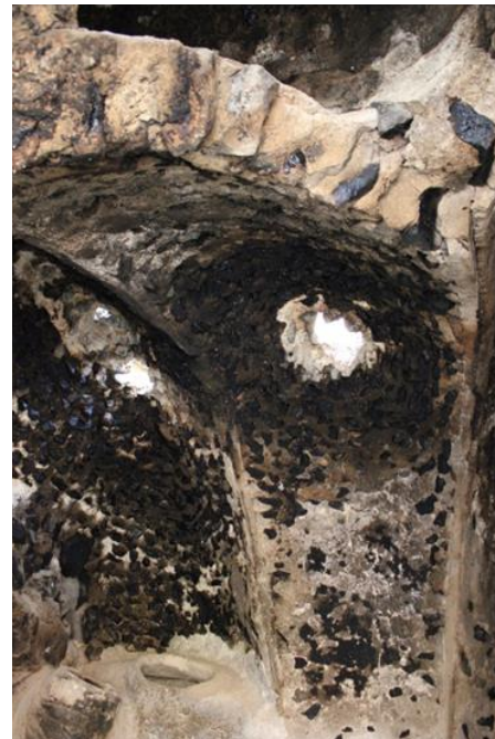
Fig.18. Stone arch and gypsum rib and middle hole
