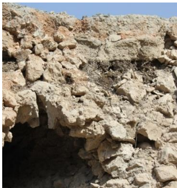
Fig.21. The four layers of roof water insulation and the arches below it are shown in the figure
