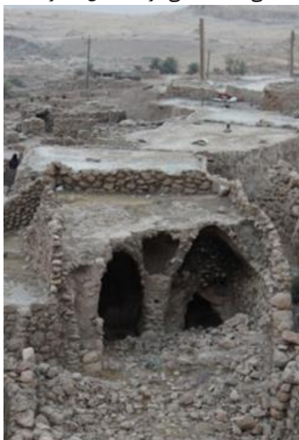
Fig.19. Small arches between two main arches
