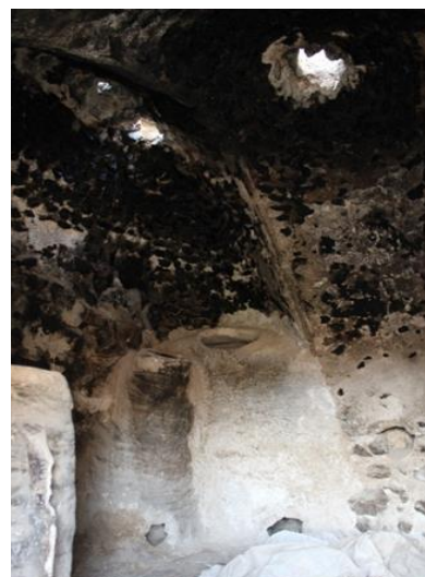
Fig.24. Two Tabos Attached together (and the roof of the arch and the rib above them)
