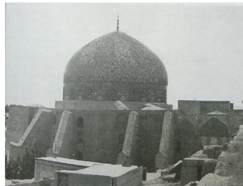
Fig.15. Addition of buttresses to Sheikh lotfollah mosque (Zander, 2017)
