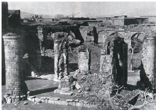
Fig.10. The ruined Khodakhane before reconstruction (Wilber, 2008)
