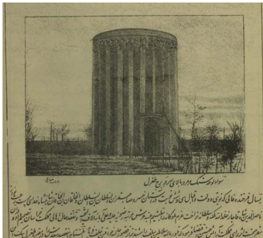
Fig.7. Before and after restoration images of Toghrol tower in the reign of Nasereddin Shah (Shararf newspaper No. 29, 1302 Islamic calendar)
