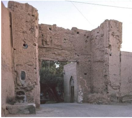
Fig.11. Darb-e-Kushk, after removing the tilework (Golombek 1976)
