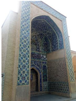
Fig.13. The present condition of Qotbie mosque portal in Chehelsotoon garden
