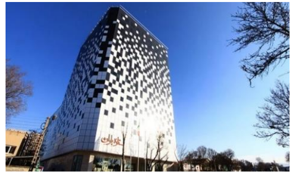
Fig. 3. Setarehbaran commercial complex
