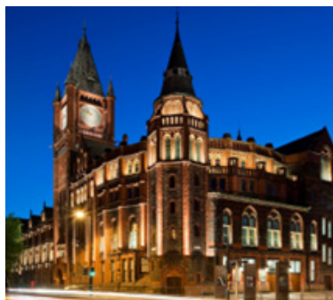
Fig. 8. Lighting of Manchester City Hall
