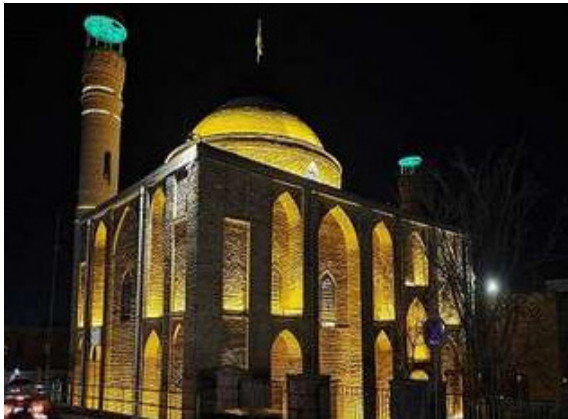
Fig. 4. Lighting of Saheb-al-Amer Mosque in Tabriz
