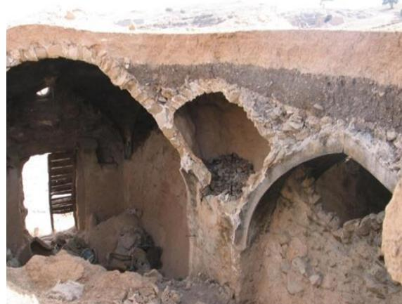
Fig.22. Layers of covering between the arch and the roof in one of the villages of Shushtar city
