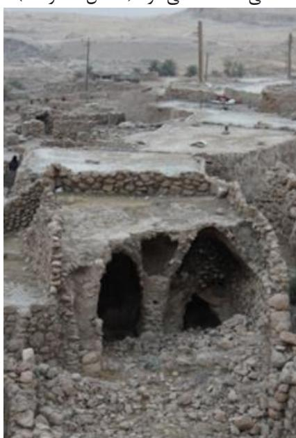
Fig.19. Small arches between two main arches
