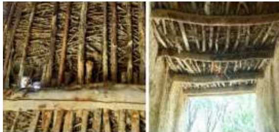
Fig. 11. Details of the roof of the Keché
