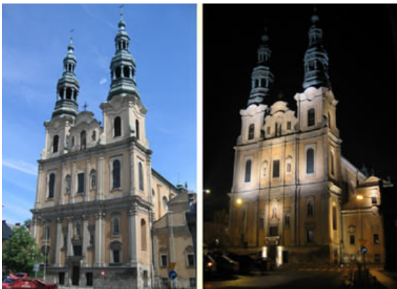
Fig. 5. Front elevation of the Church of St. Francis, day and night views (Górczewska, 2011)
