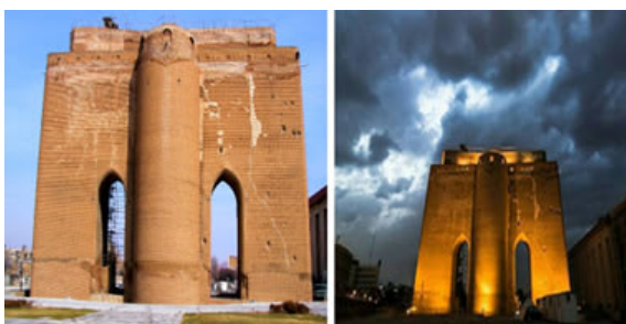
Fig. 6. Lighting of Arg-e Alishah of Tabriz, daytime and nighttime views
